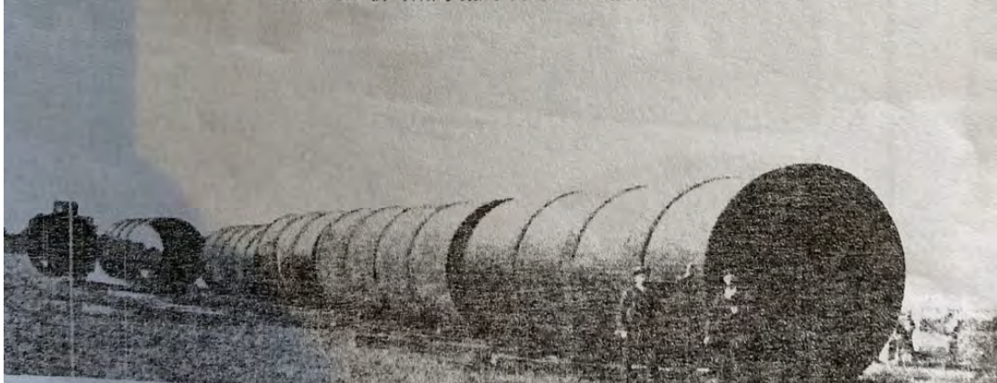
SECTIONS OF THE FIRST KILN AWAITING ERECTION
